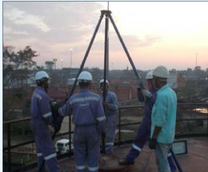
Photo 2: Support Erection for launch of rover
